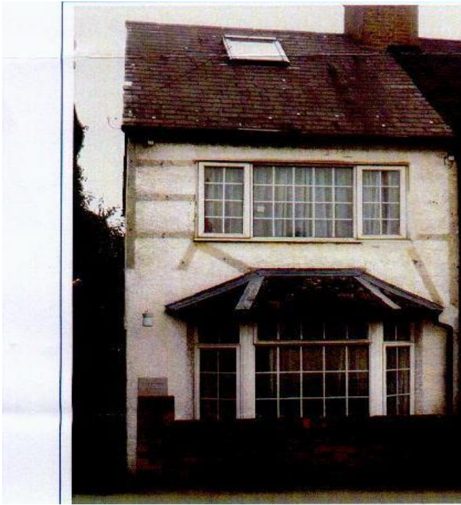
Fig. 6. Ledgers Road, Slough
